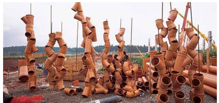
Art in construction: the wide range of pipework will be pre-graded
